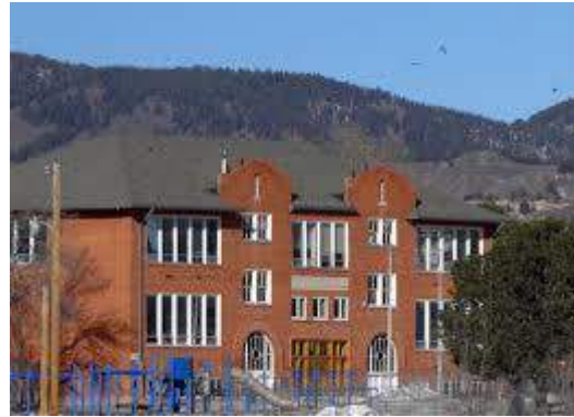
Lewis Palmer D-38 Administration building (a.k.a. Big Red) 146 Jefferson Street, Monument, CO 80921. Please use the West or North entrances!
