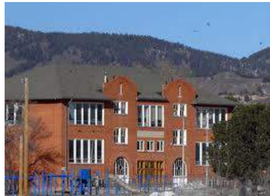
Lewis Palmer D-38 Administration building
