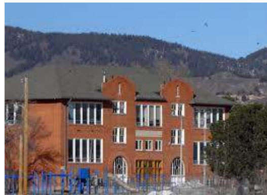
Lewis Palmer D-38 Administration building
