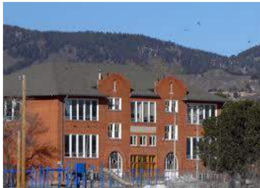
Lewis Palmer D-38 Administration building
